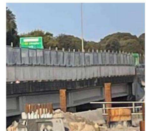
Cam River Bridge
