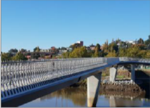
Pedestrian & Cycle Bridge + Northern Car Park $10m 2019 - 21
