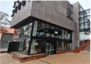
Podium building (fit-out) $2.7m 2019 - 21
