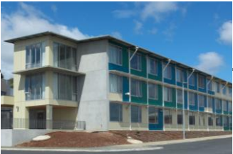
Student Accom West Park Apartments $7m 2014 - 15
