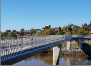
Pedestrian & Cycle Bridge + Northern Car Park $10m 2019 - 21
